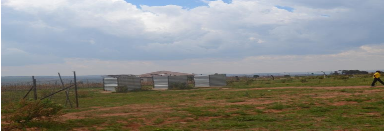
Figure 3: Toilet structures at Tjetje Technical high School
